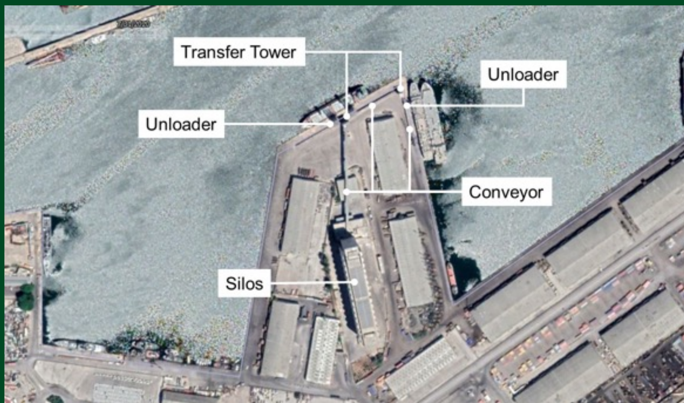
Figure 2: Port of Beirut grain import facility
